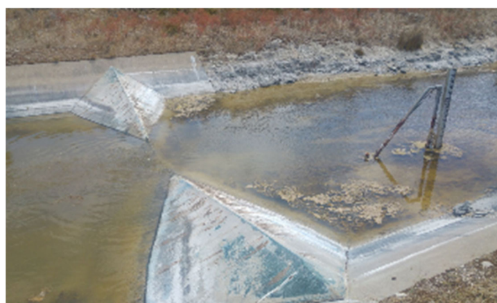
Figure 3.2. Crump weir gauging station for water levels within Salt Creek.
