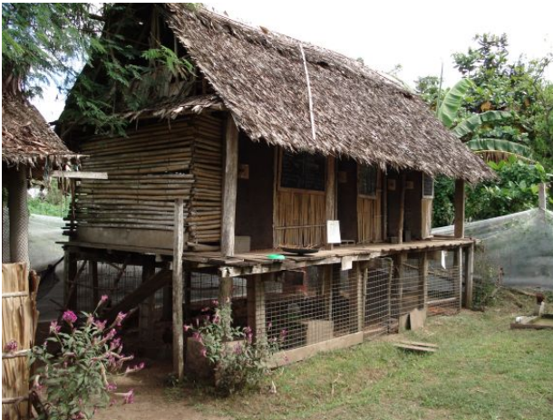
Kastom Gaden poultry feeding demonstration facility in Solomon Islands
