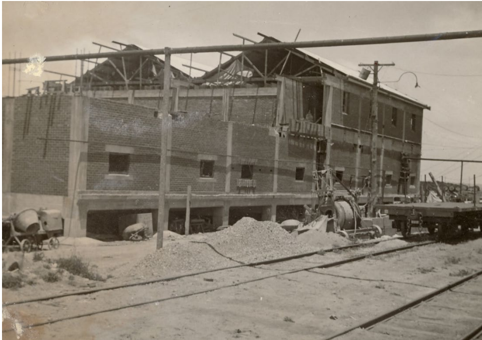
Major extensions to abattoir and freezer facilities under construction at Pt Lincoln 1941.
