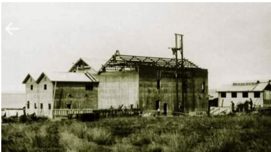
Early construction of the Port Lincoln abattoir complex c1924
