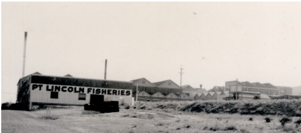
Fish cannery building at the Port Lincoln Abattoir c1940s.
