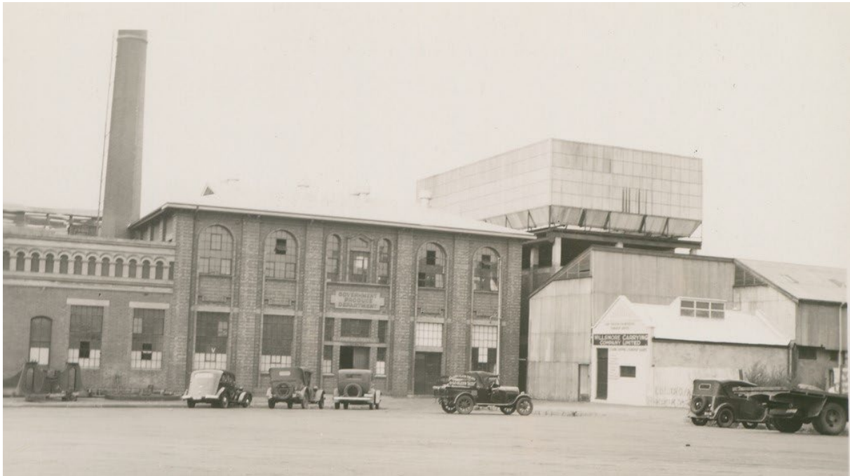
Government Produce Department Light Square facilities and head office in 1942 showing the large cooling tower for the refrigeration plant on the right. The two-storey office block in the centre of the photo was built in 1926-27. Source: State Library of South Australia; Image B 10905. Other photos in this series include B 2994 (1925), B 8838 (1925).
