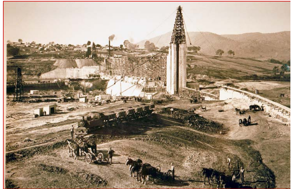
Under construction, 1928 – using horse-drawn trolleys and drays
