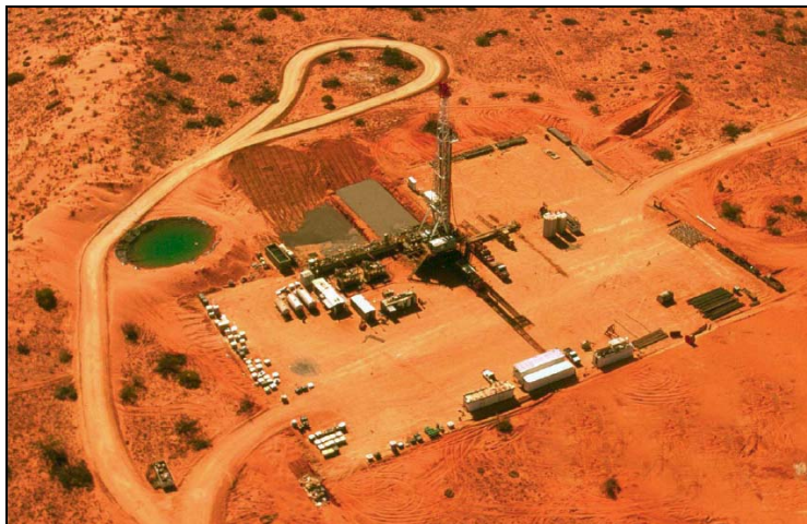
Plate 1: Petroleum exploration drilling showing typical layout of well lease
