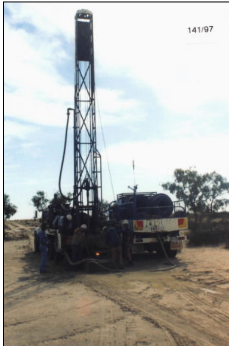
Plate 3: Typical Up-hole Drilling Rig
