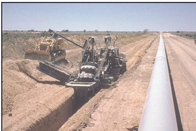
Construction of Della trunkline. (Photo T15557)
