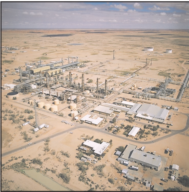
Moomba processing plant, Cooper Basin. (Photo 43803)
