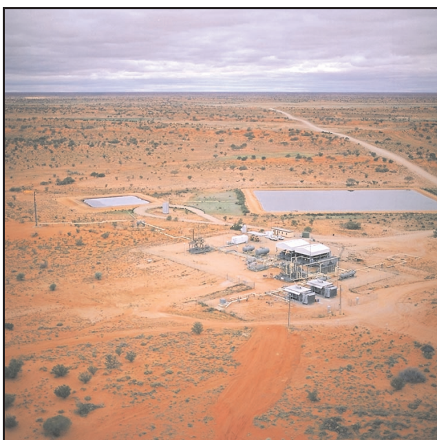
Cooper Basin satellite facilities. (Photo 43790)
