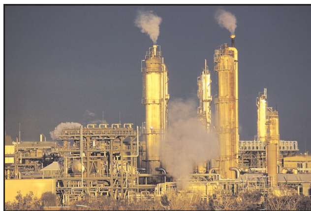
Carbon dioxide removal towers, Moomba. (Photo 43373)
