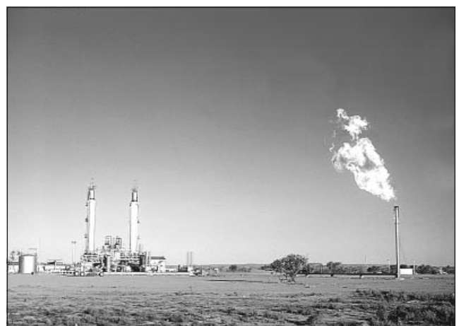
Moomba natural gas processing plant, November 1969. (Photo 43830)
