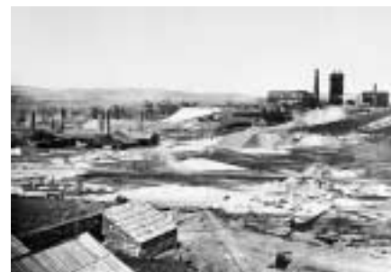
Henderson Plant at the Kapunda Mine, 1875. (Photo N024003)
