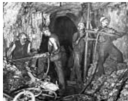
Drilling blast holes with jackhammers in a slope at Wallaroo Mines, ~1916–18. (Photo N010765)
