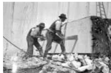
Hand sawing of a toppled pillar of Gambier Stone in 1950. Note solution cavities and root holes. (Photo N008585)
