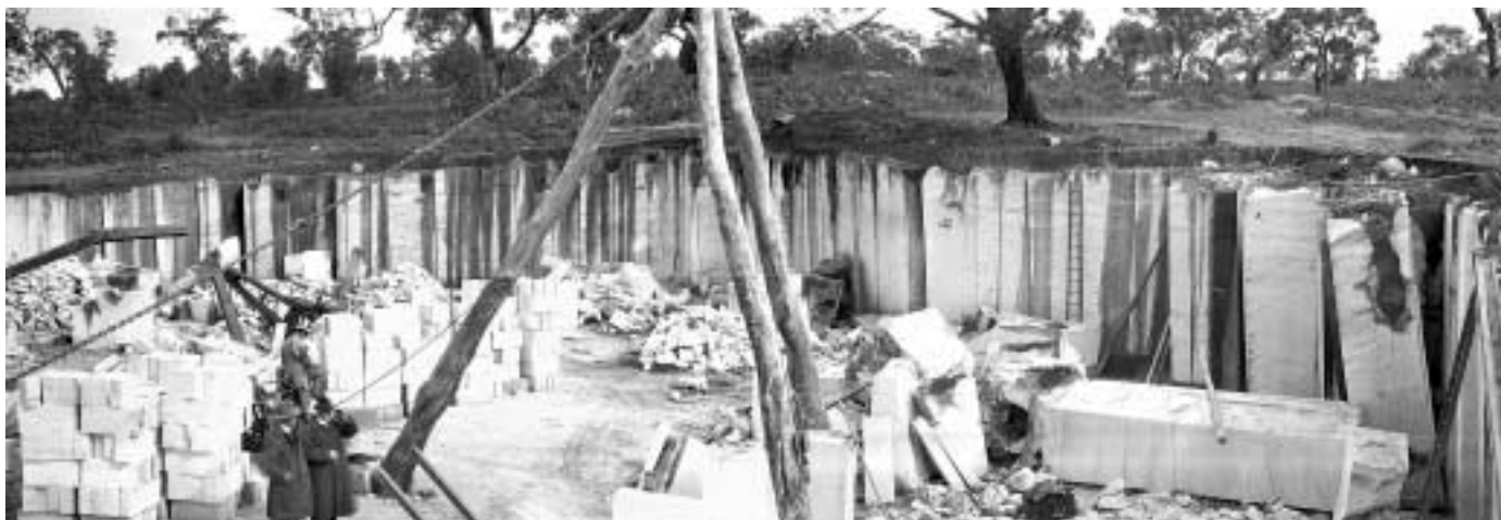
Quarry near Mount Gambier in 1920 showing hand-sawn faces in background, toppled pillars in right foreground and stacked ashlar of Gambier Stone at left. (Photos N000471, N000472)
