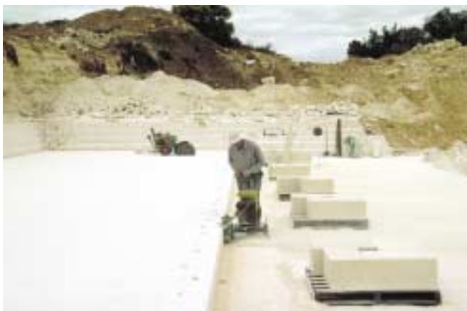
Block sawing in 1986 using self-propelled, petrol-driven Ploenges saws, Steely Quarry near Mount Gambier. (Photo 038199)
