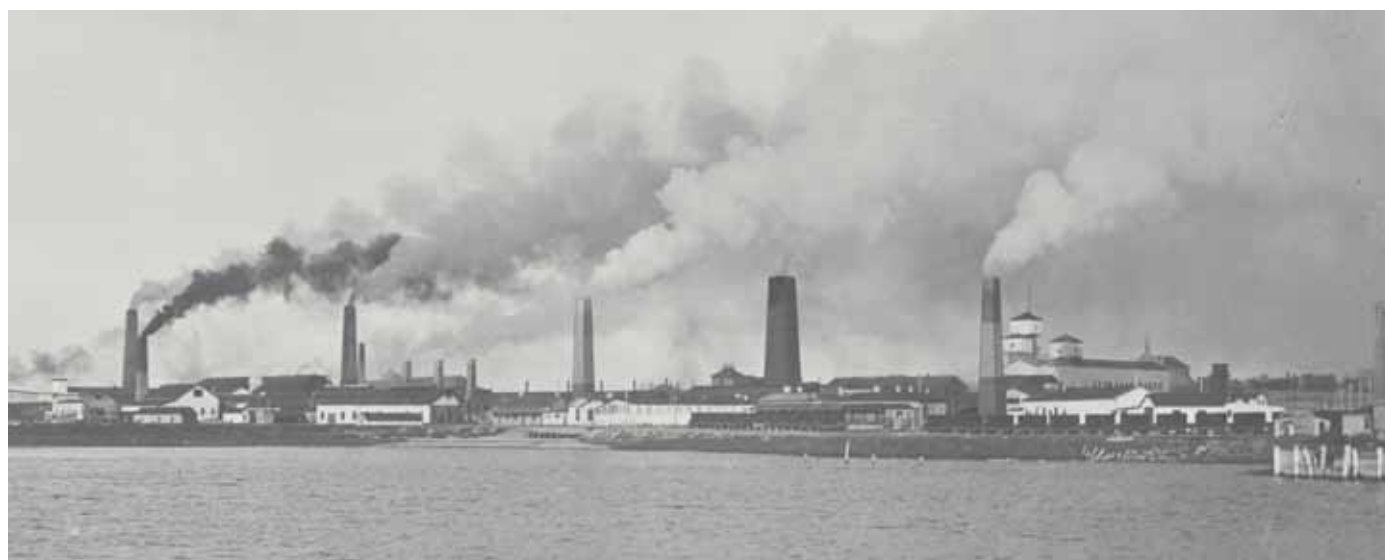
Wallaroo Smelters viewed from the Wallaroo Jetty ~1910. The plume of sulphur and carbon-rich smoke was seen for kilometres, and became a well-known landmark. Hughes Chimney Stack is the black, widest chimney near the centre of the image. (Photo N10758).
