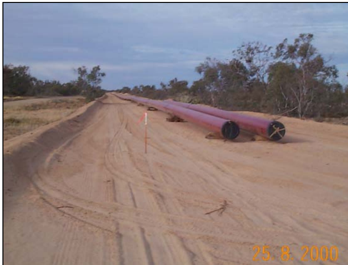
Plate 5: Welded pipe string with end caps
