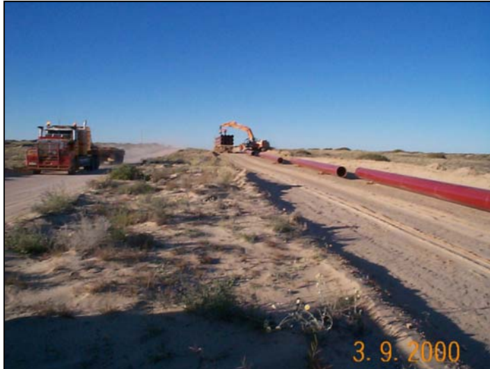
Plate 4: Unloading and stringing pipe
