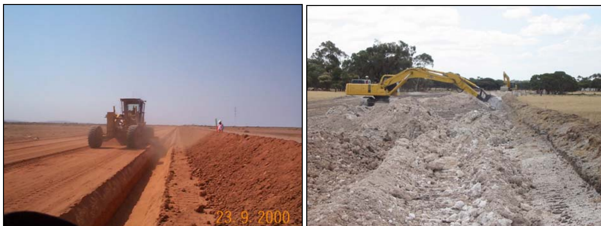
Plate 7: Backfill with a grader or excavator
