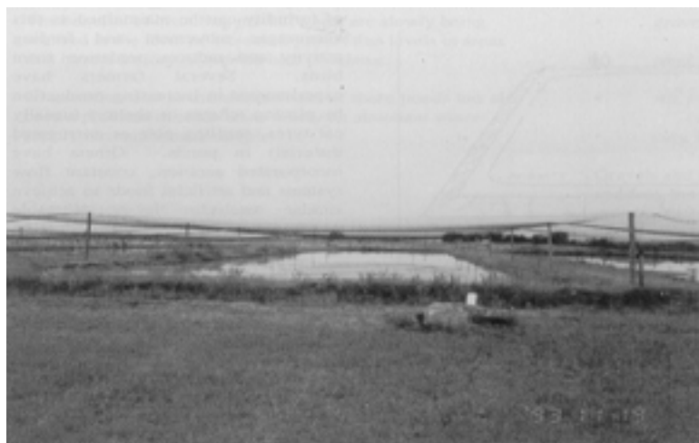
Pond covered by bird netting supported by pine poles.
