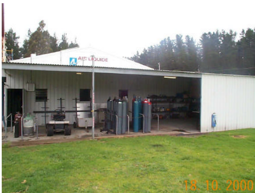
Plate 2: Contained storage area.
