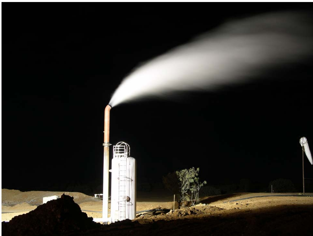
Figure 2: Habanero 2 Steam Separator. The well flowed at 25 L/sec with a wellhead temperature of 210°C during testing in May 2005. Photo courtesy of Geodynamics.
