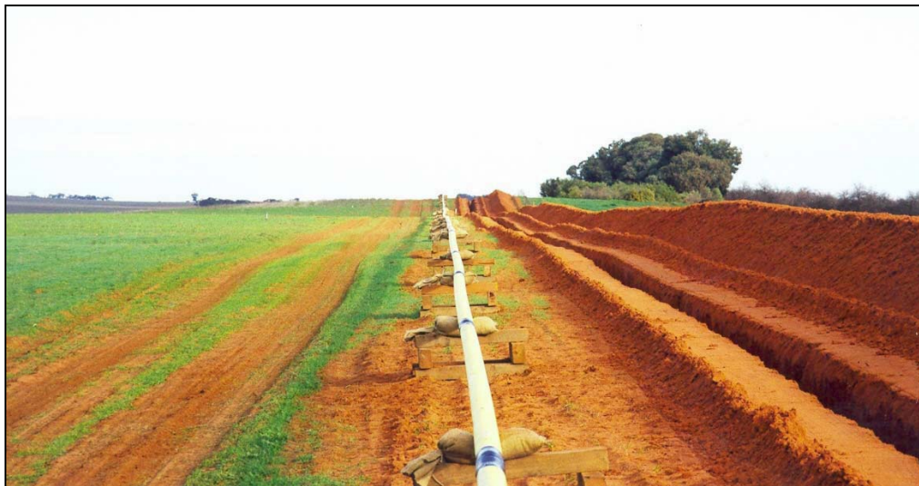
Plate 3-4: Welded small diameter pipe ready for lowering-in
