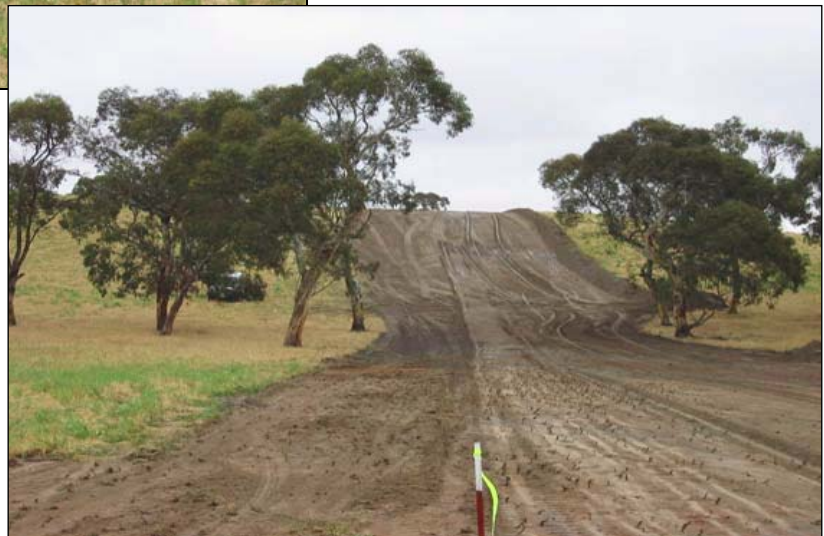
Plate 3-1: Clear and grade (before and after)
