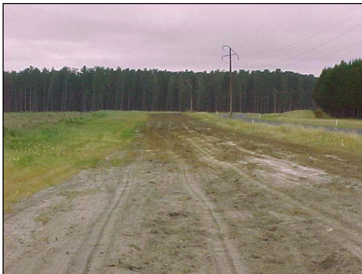
Plate 3-7: A newly reinstated easement
