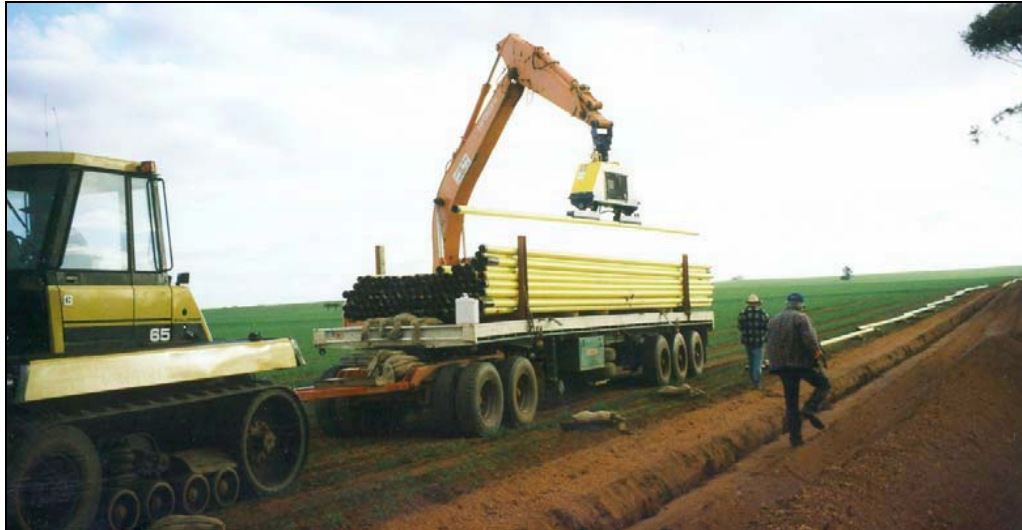
Plate 3-3: Stringing a small diameter pipe
