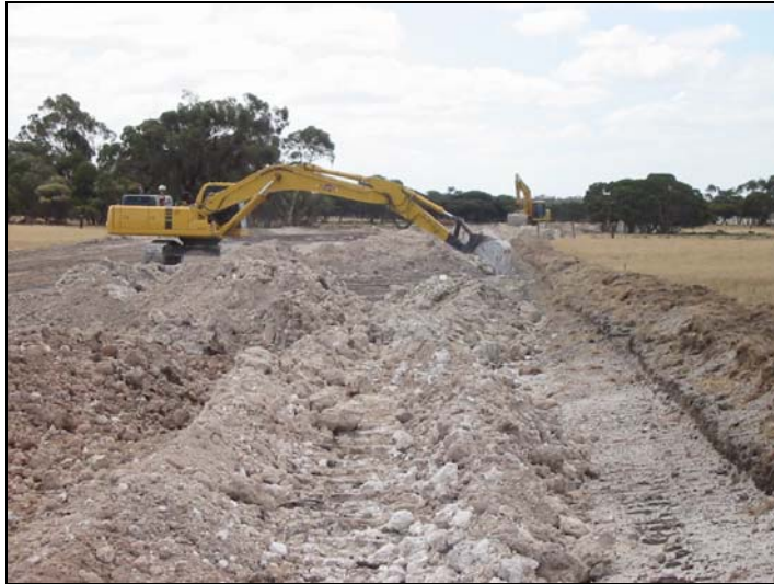
Plate 3-6: Backfill
