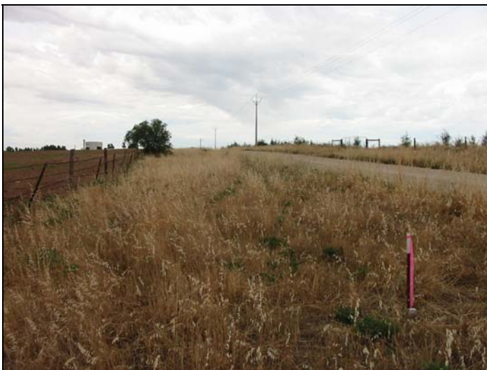
Plate 2: Pipeline alignment showing vegetation in road reserve, facing south-west
