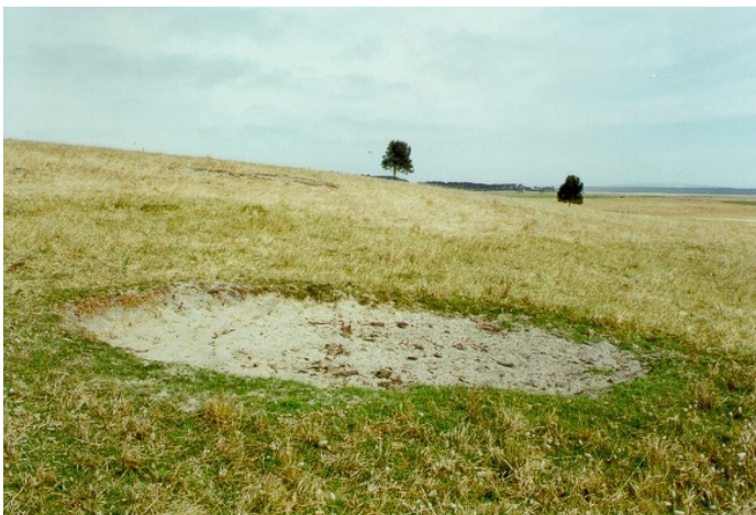
Figure 6. Close up of existing erosion. No activities will take place on the dune due to the sensitivity to erosion once the sand is disturbed.
