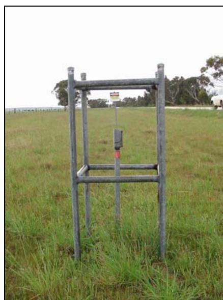
Pipeline Marker and Cathodic Protection site
